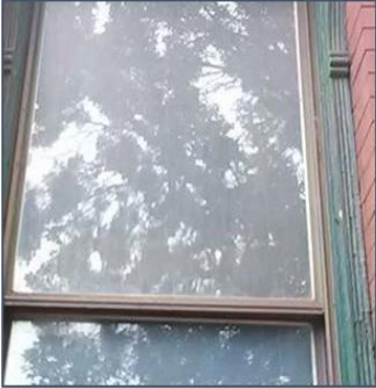
Repairs are complete
