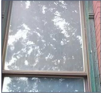
Repairs are complete
